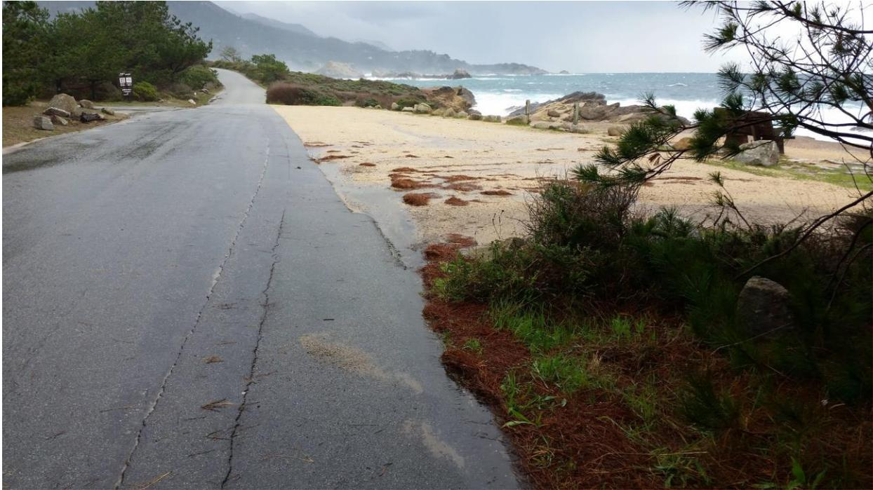
**Figure 29: Water running down the road into the Piney Woods beach parking area. This increases the rate of bluff erosion by directing runoff onto the devegetated parking lot and bluff.**
