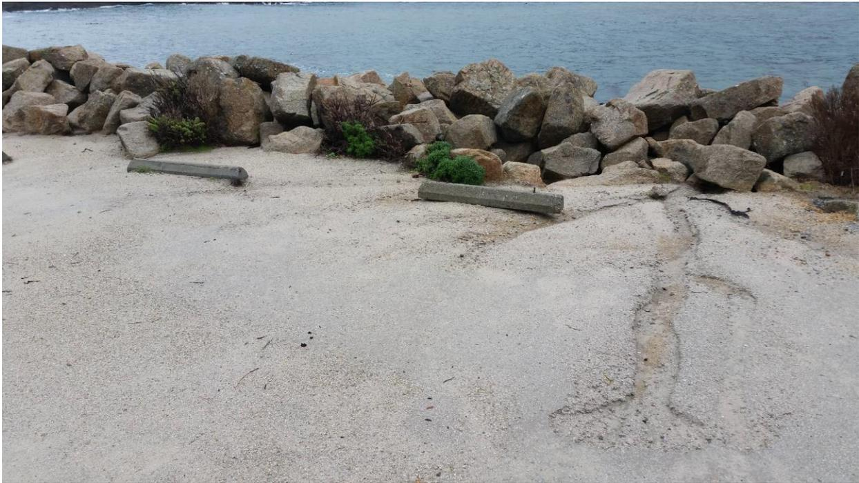
Figure 34: Erosion of the Whalers Point parking area into the ASBS.
