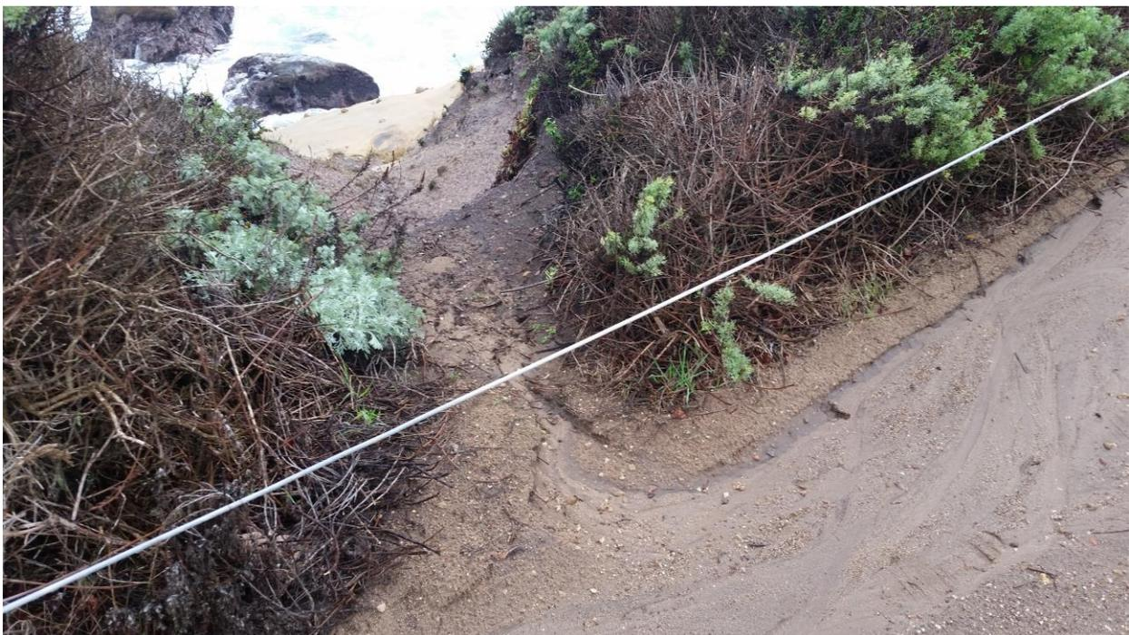
**Figure 28: UCT off of trail by Sand Hill Cove allowing for sediment to discharge directly into ASBS.**
