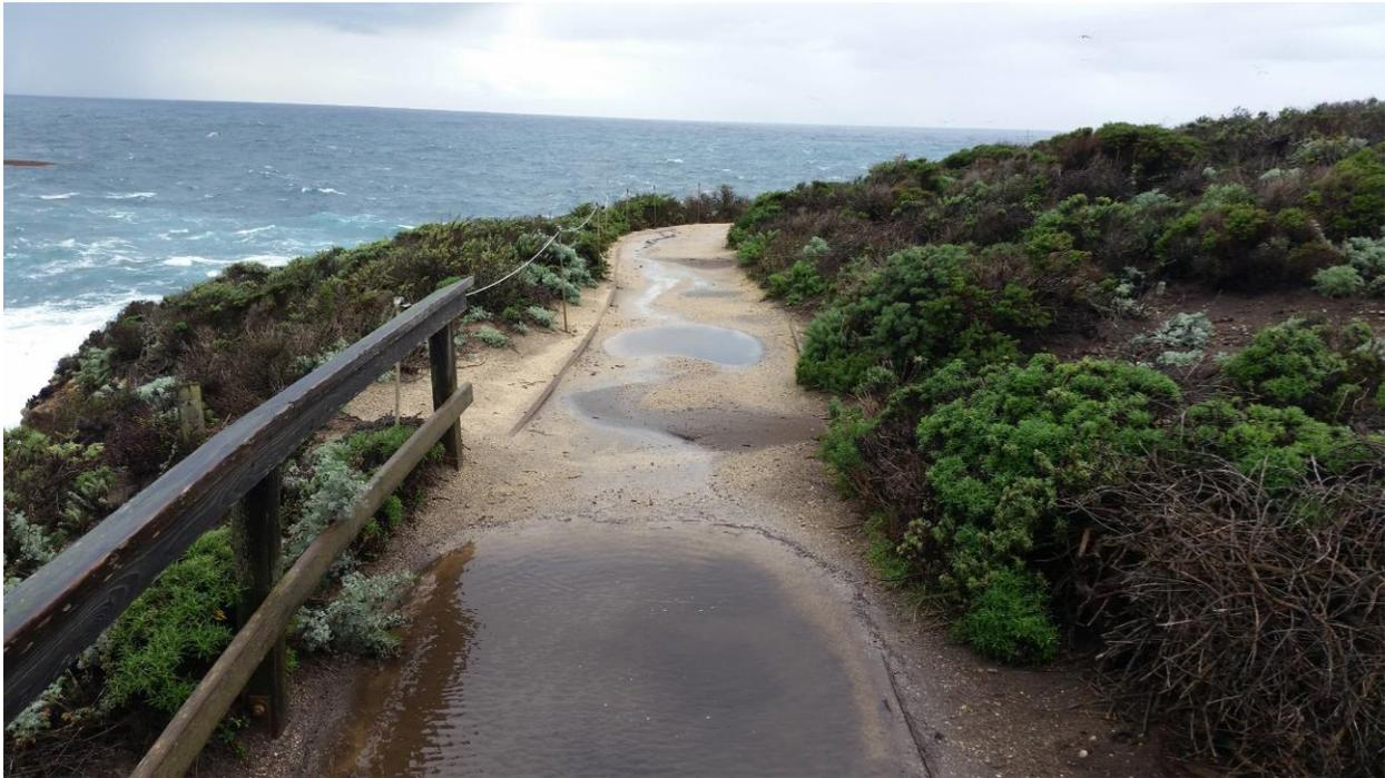
**Figure 27: Ponding and running water on Sand Hill Cove Trail. Lack of water control features leads to sediment transport and trail degradation.**
